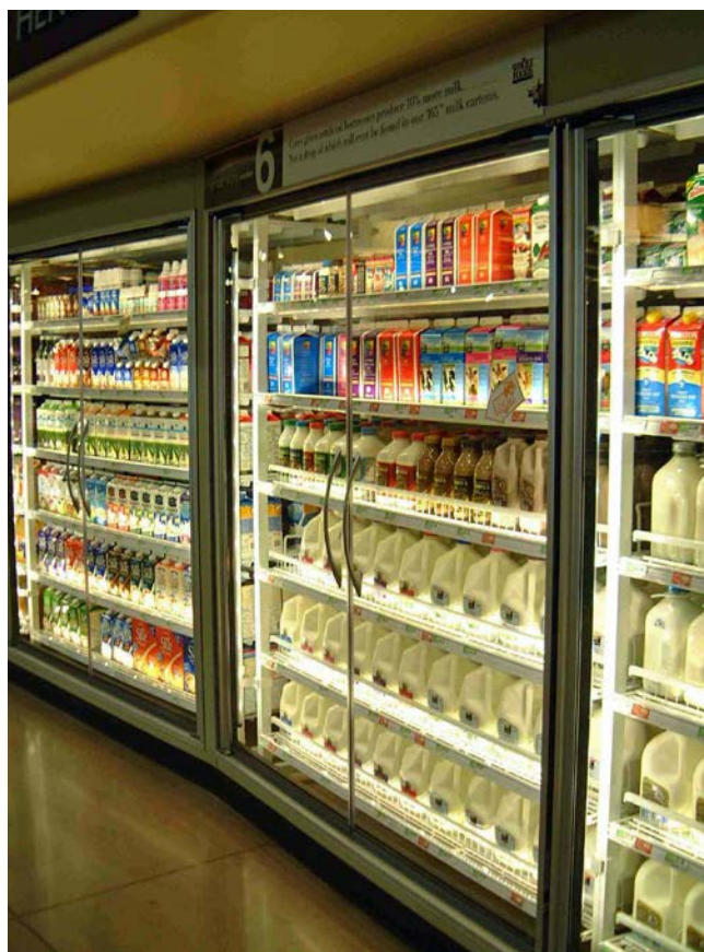
Figure F-3 Doors installed on medium-temperature refrigerated cases at a Whole Foods Market
