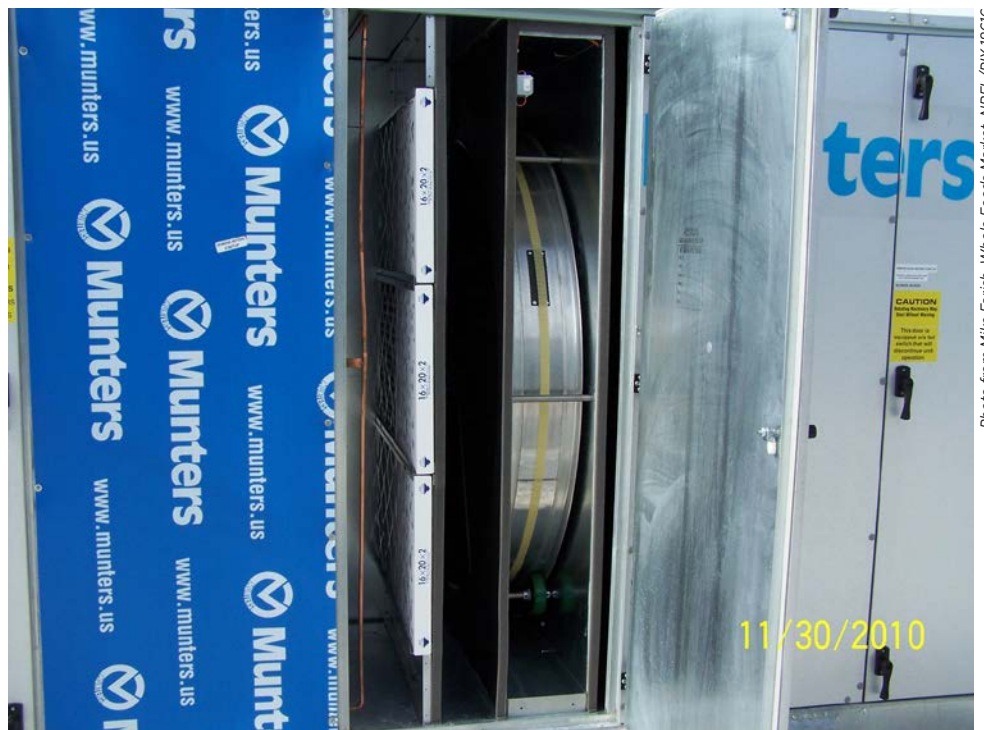
Figure F-4 Desiccant wheel used for dehumidification at a Whole Foods Market
