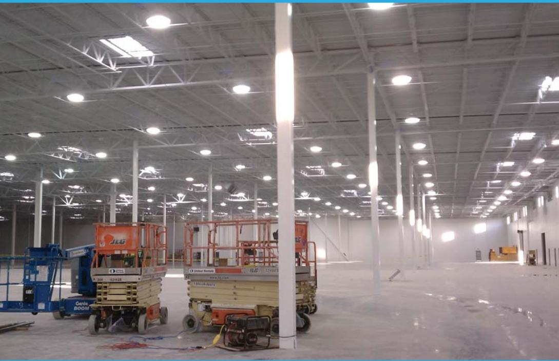
Induction lighting technology is a proven solution for an efficient building energy strategy. Induction bulbs radiate soft, pleasant light with minimal glare and peaks. Longer bulb life-spans drastically reduce maintenance costs by lowering expenses for parts and labor.
